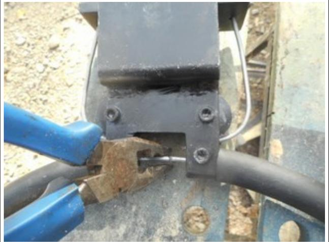
Minimise the gap between the wires.
